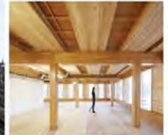
CLT (Austrian) with 150mm cement core access floor system
