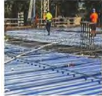
200mm post-tensioned 32MPa 50% fly-ash on 25% recycled bondek.
