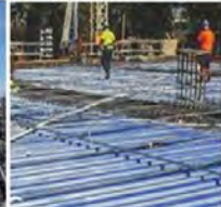
200mm post-tensioned 32 MPa on bondek.
