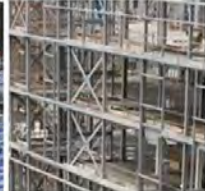
Composite steel frame 200mm thick 32 MPa slabs on Bondek
