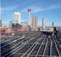
200mm post-tensioned 32 MPa on formply.
